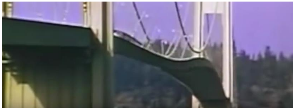
Tacoma Narrows bridge displaying aeroelastic flutter, which may not technically be resonance, depending on how you define resonance.
